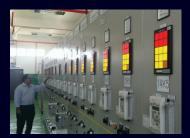
Sequence test capabilities where all windows light up to allow operator to easily check annunciator operational health.
